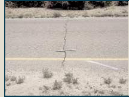
Transverse Cracking
