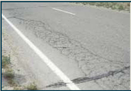
Alligator Cracking
