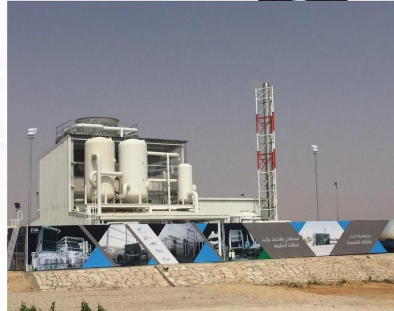
The commercial pilot at Solar Village of 75 m<sup>3</sup>/day and 2 MW cooling, built jointly by KACST\_MEDAD\_KAUST, treating the RO rejects.
