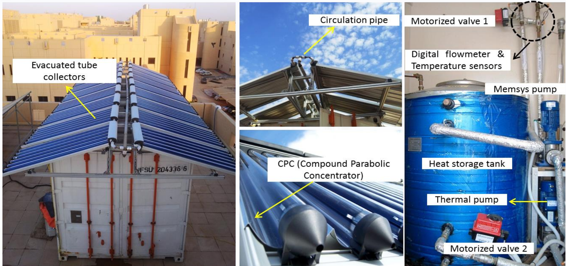
Figure 14. Overview of solar thermal system
