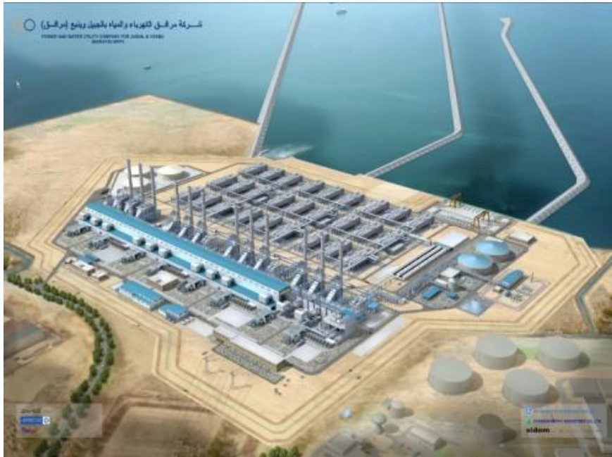
Figure 3. Desalination plant in Saudi Arabia
