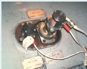
Figure 1 Vibration transducer on turbine: labelled and appearing to be 'Bearing Vibration'
